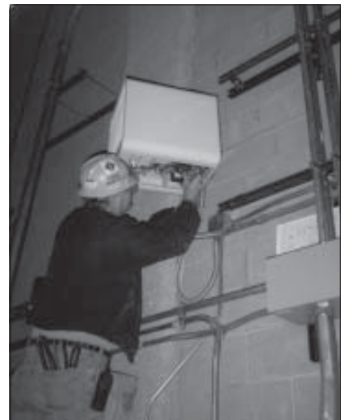
A unit heater being installed in a Chicago high rise electrical room for humidity and freeze protection.
