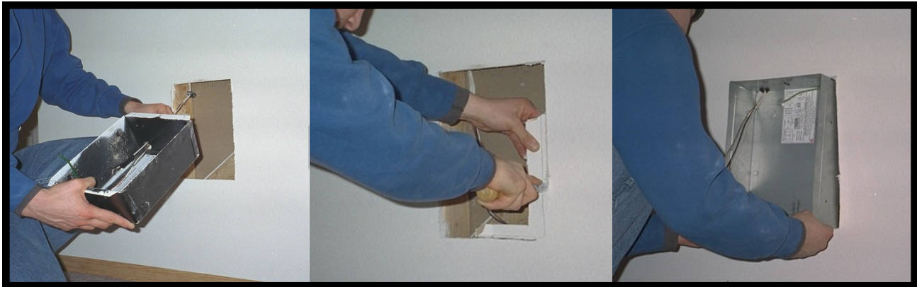
Apply power wires with grommet and ground wall box. Insert into wall leaving 1/2 inch
