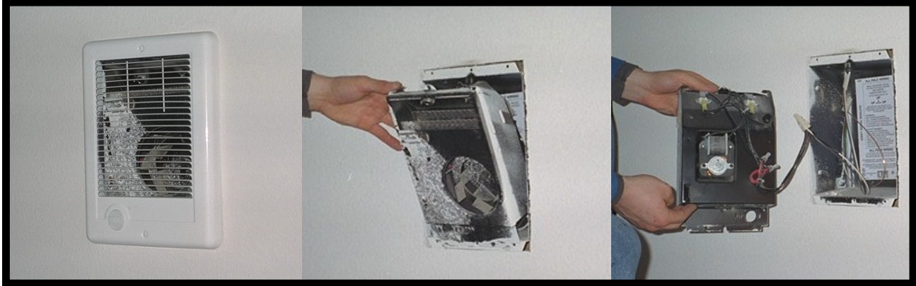
Remove wire nuts from interior.
