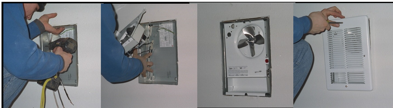
Attach can to stud on one side and use 2 screws just behind the wall board to prevent the other side from moving forward.
